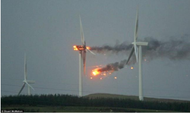
Wind Turbine Fire in Ayrshire Scotland
